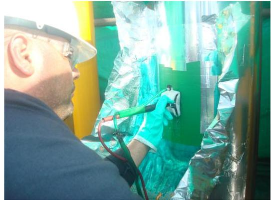
When undertaking the repair work, two SIFCO ASC technicians were situated near the top of the derrick, 450ft in the air, to perform the repair. It took them a total of 24 hours to complete the work and return the platform to full operation, as opposed to three months to replace the shaft.
